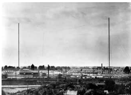
5XX Long Wave transmitting aerials (1927)
