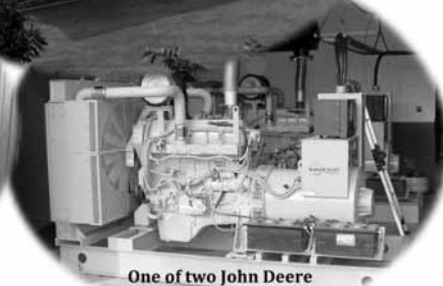
One of two John Deere 300 KW Generators
